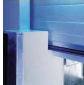
Gap for the sectional door.
