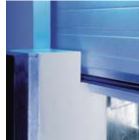
Gap for the sectional door.
